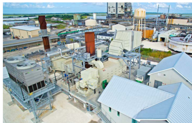
Figure 4. The Eight Flags Energy Plant, Florida Public Utilities. Source: Cottle Communications
