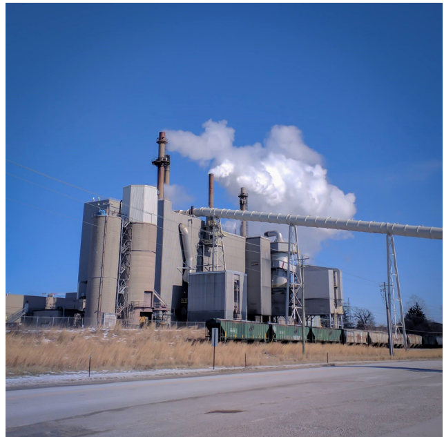
Figure 7. The Wade Utility Plant, neighbor to the planned Purdue CHP plant site.
